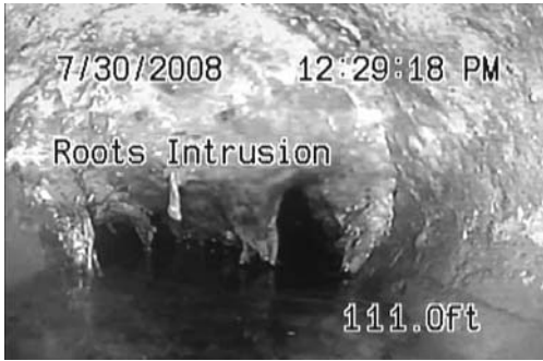
Figure 21 – Display Screen with Slide Text, Time and Distance Shown (Distance measured from system zero-point)
