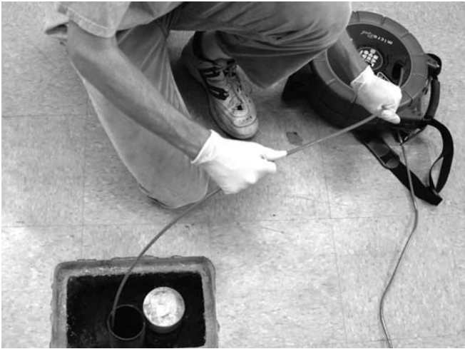
Figure 25 – Allowing cable to loop may kink the cable while pushing into drum
