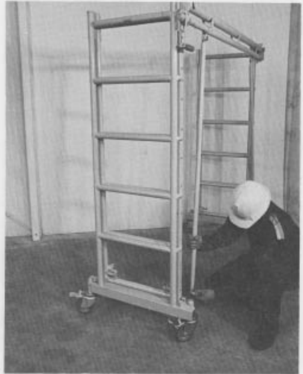
Jog base of end sections to facilitate brace pin alignment
