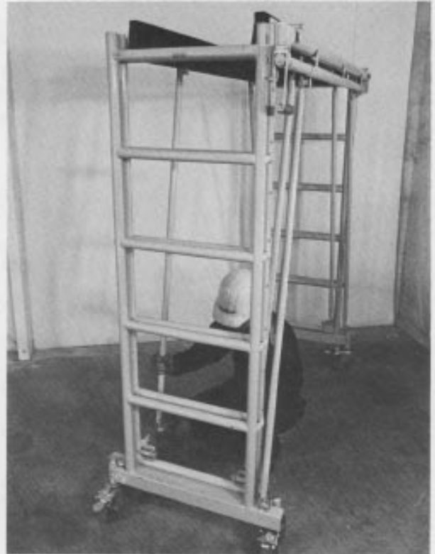
Attach deck braces to telescoping ladder sections. Jog base of end sections to facilitate brace pin alignment.
