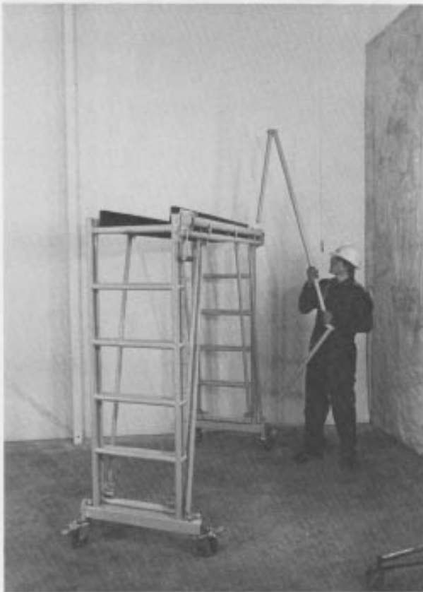
Guard rails are lowered into top end of telescoping ladder sections. CAUTION: KEEP FINGERS CLEAR OF HINGE JOINTS WHEN HANDLING GUARDRAILS.
