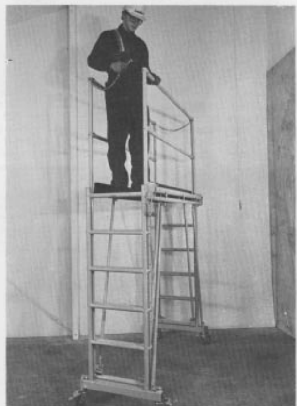
Attach safety chains between top rails on each end.
