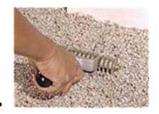
• If there's a patch that needs to be replaced, make sure you have enough replacement carpet with the grain or pattern going the right way. Cut out the bad section of carpet, lay in seam tape and follow the previous steps.
