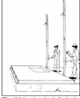
The lift begins, both Jacks being operated in unison. (If one worker is top edge of the wall during the entire raising the wall, he simply moves from one Jack to the other, avoiding excessive twisting of the wall.)
